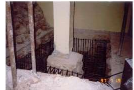
hardening the surface and installing the dowels.
