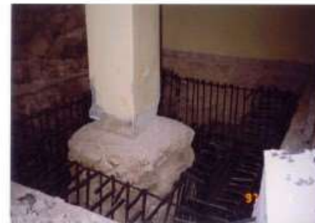
Photo 15. Installing the main steel.
