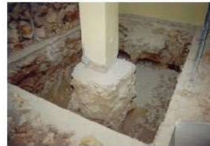
Excavating around the footing.
