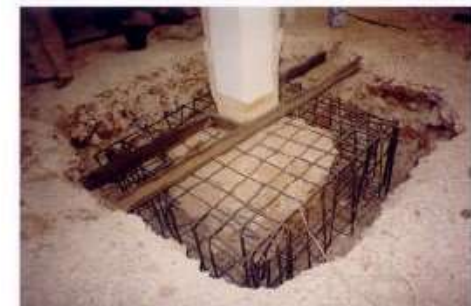
Photo 16. Completing the jacket.
